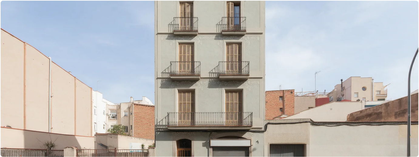
Carrer de Verdi 31 — twenty-four flats over the shuttered pharmacy.
